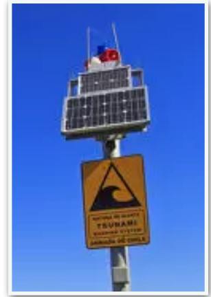
Tsunami warning alarm in Patagonia, Chile.
