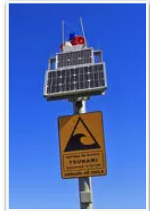
Tsunami warning alarm in Patagonia, Chile.
